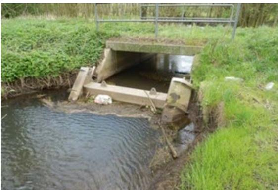
Technical installation for the retention of floatsam, not to be mapped as construction
